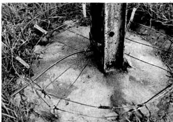
The base of the cage unipole, showing the method of terminating the radial wires.
